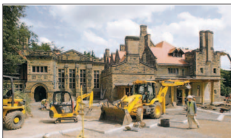
Work in progress at the hotel
